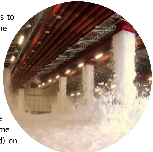
Fig. 2 Fixed foam fire-extinguishing system
